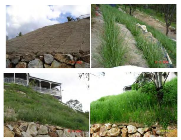
Rehabilitation of a very steep and erodible slope resulting from a landslip following heavy rain in Australia
