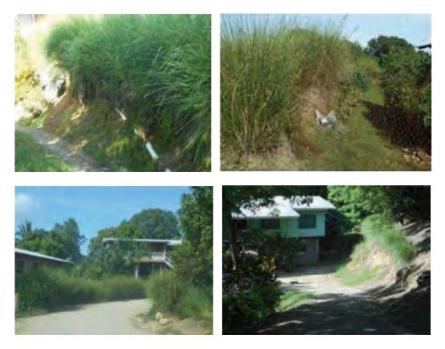
**Pictures 11 – 14:** Vetiver planting on cut batters to protect slopes on residential properties.
