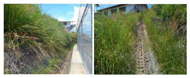
**Pictures 7 & 8:** Virtually silt free drains demonstrate effectiveness of Vetiver in reducing erosion
