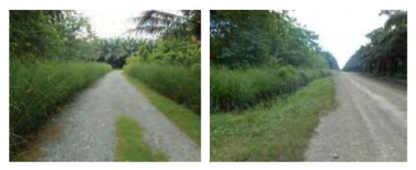
**Pictures 34 & 35:** Plantation road stabilization, also planted to stop debris from being washed onto the roads during flooding.
