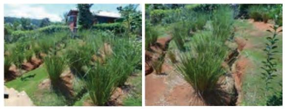
**Picture 21 & 22:** Vetiver planted in front of drains which were dug initially to reduce velocity of water to control soil erosion on hill top.
