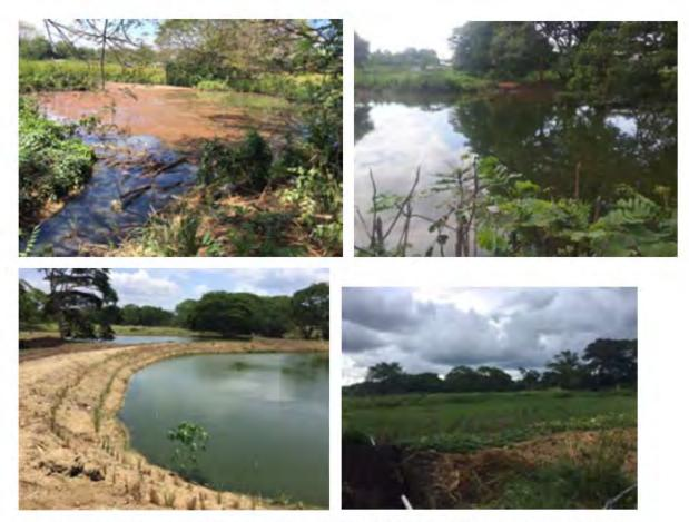
Fifteen thousand vetiver slips planted on 3,000m<sup>2</sup> treat 2,186L/day sewerage effluent.
